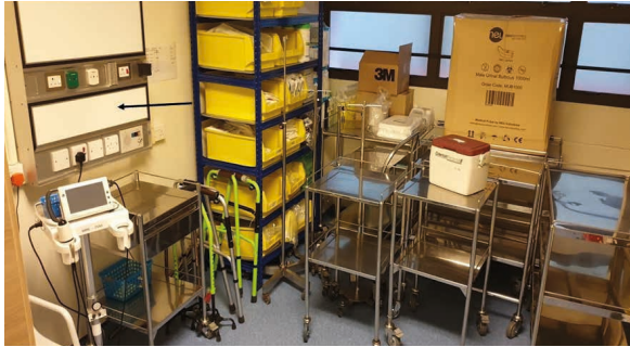
Figure 2 The treatment room within ward 42 where catheter insertions and renal biopsies were performed. It has been converted to a storeroom. The original electrical, oxygen and code blue panels (black arrow) were not dismantled.
