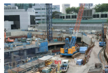
When excavation reaches basement 4, casting of the basement 4 slab will start.
