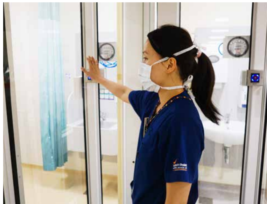
▶▶▶ Dr Tan Zihui, Associate Consultant, Department of Anaesthesiology, SGH, enters an ICU fitted with the SG-SPARC system through no-touch motion sensor doors. These doors are a unique feature of the SG-SPARC.
